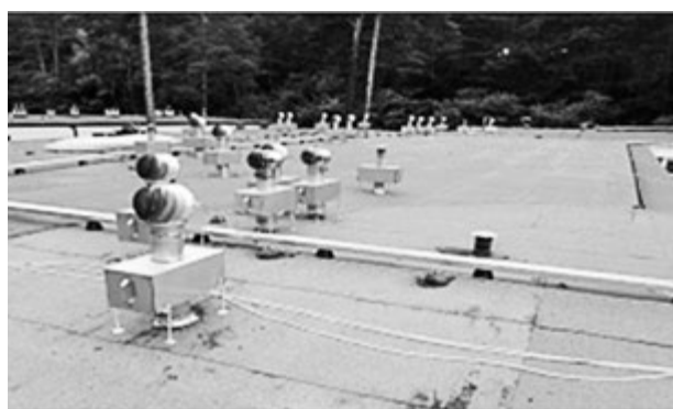
Fig 3. Ventilation stacks on the roof of the Tuberculosis Unit building
